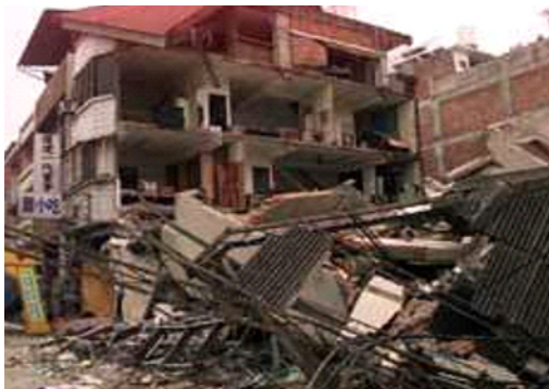
Fig. 1. Seismic damage on low-story building by big earthquake of Han-Shin area in Japan, January 17, 1995.
